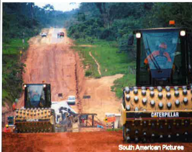
Photo 1 Road foundation preparations.
